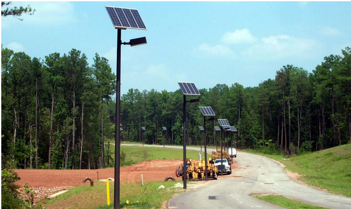
Figure I-7 CSPV: Off-grid solar lighting
