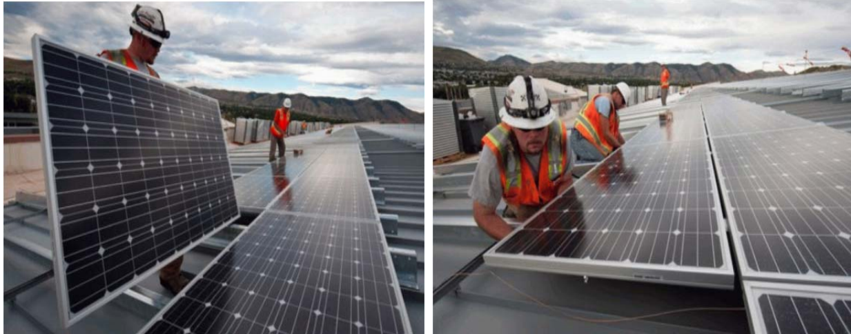
Figure I-14 Installation of a nonresidential CSPV system
