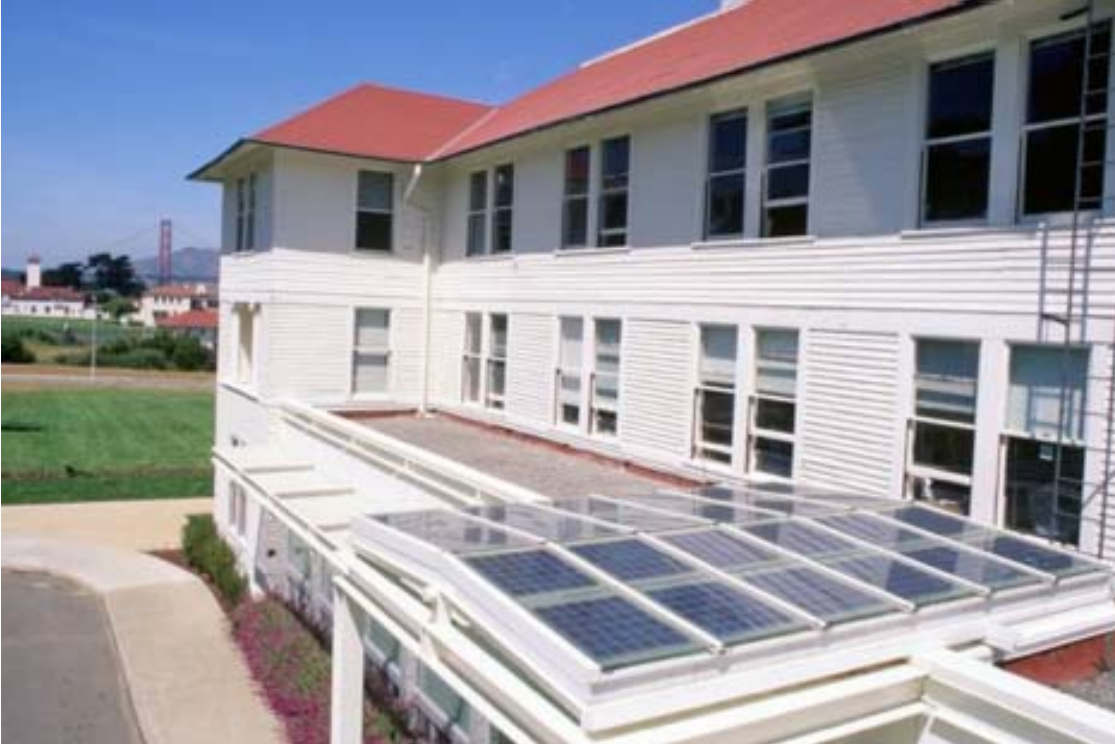
Figure I-6 Building integrated CSPV
