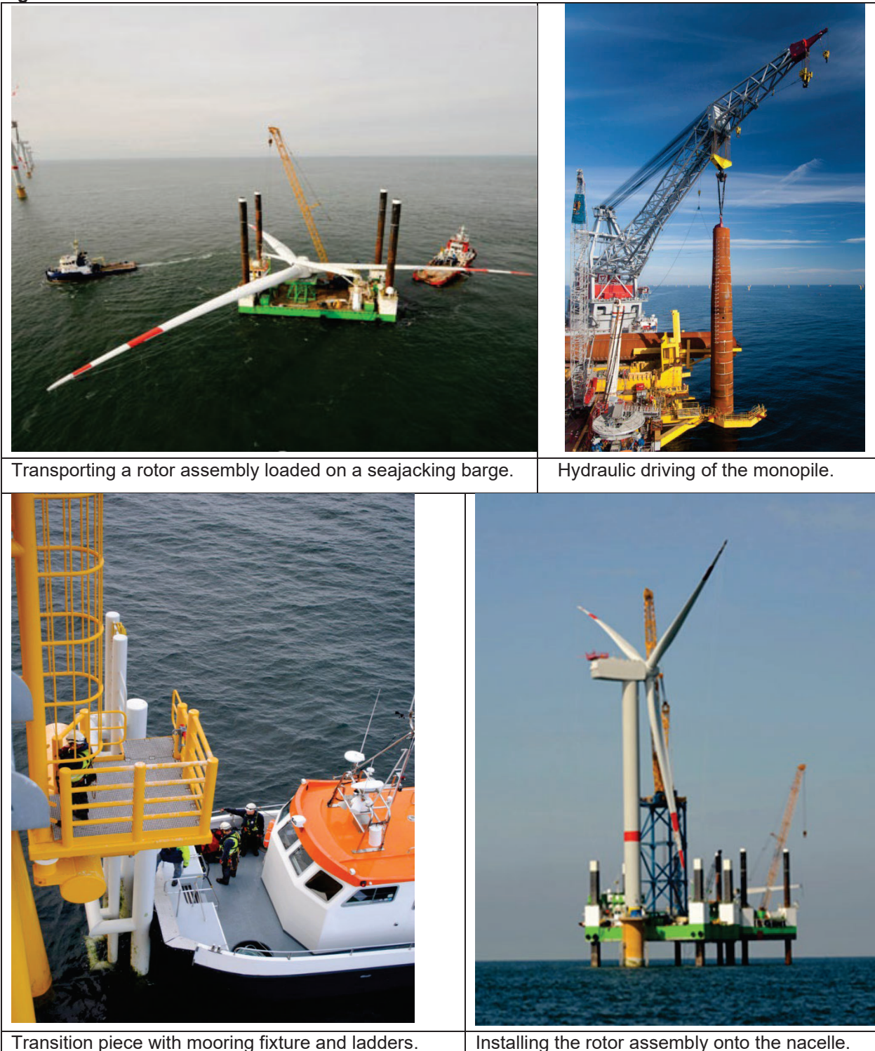
Figure 1.10 Wind towers: Turbine installation offshore
