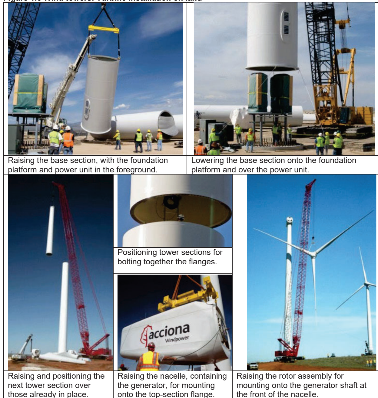
Figure 1.6 Wind towers: Turbine installation on land
