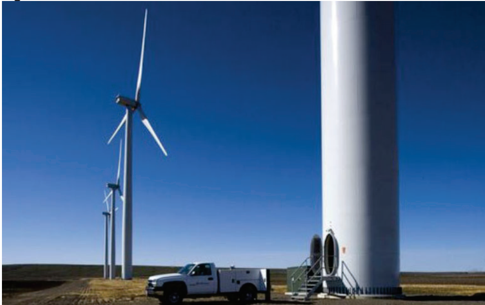
Figure 1.3 Wind towers: Installed wind turbines
