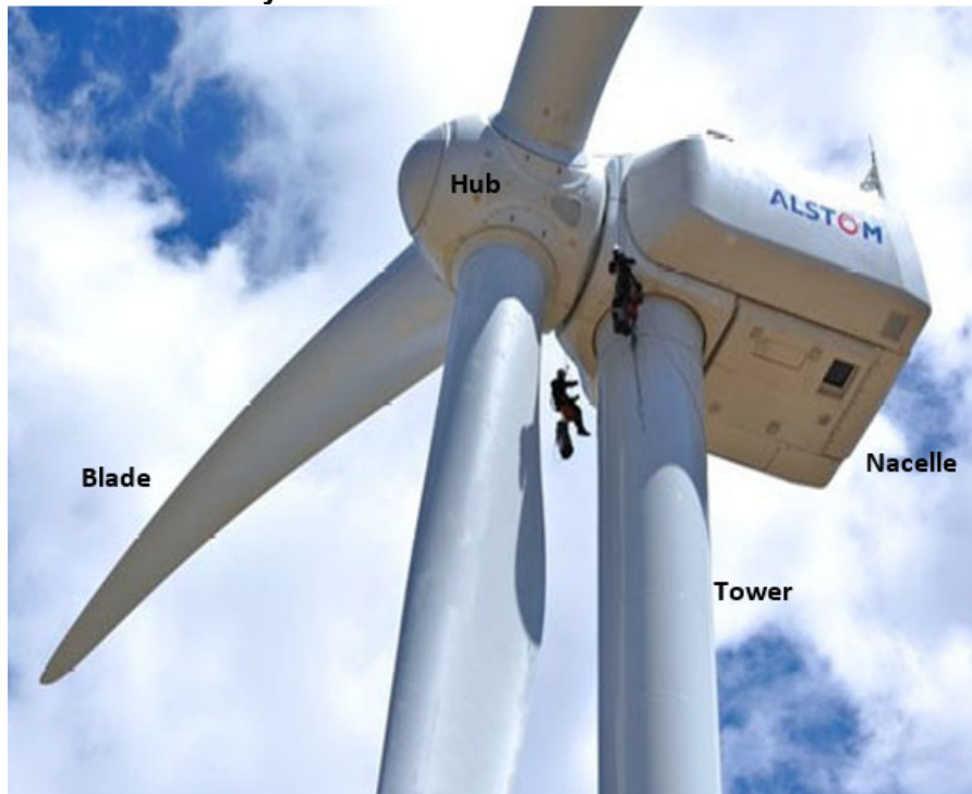
Figure I-1 Wind towers: Utility-scale wind turbine
