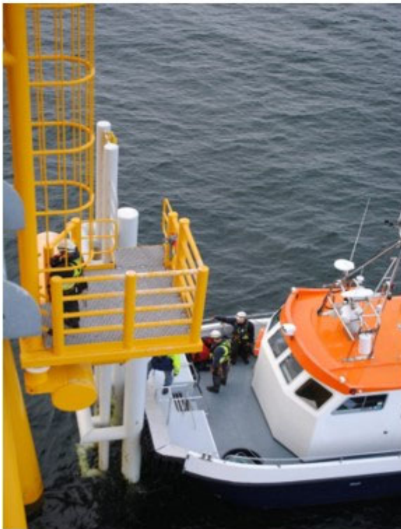
Transition piece with mooring fixture and ladders.
