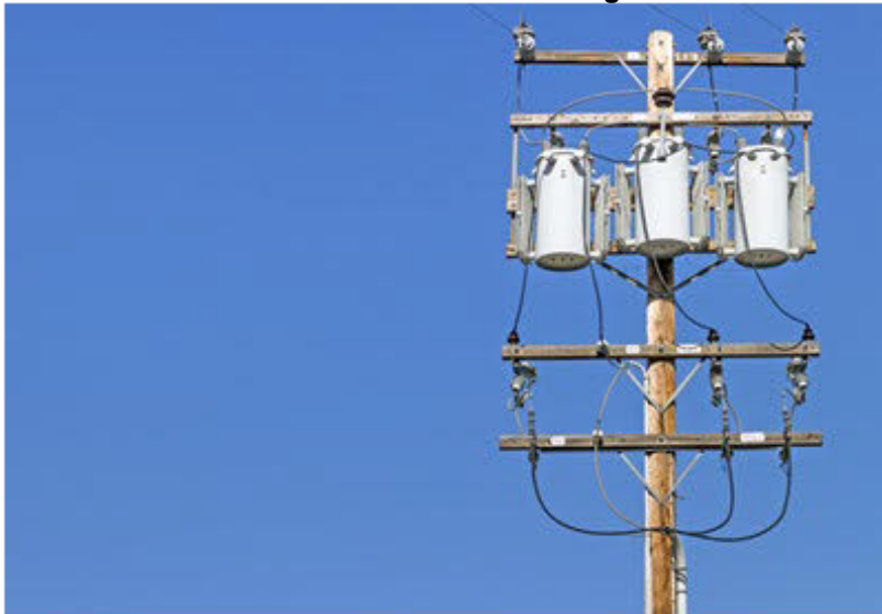
Figure I-5 Wound-core Distribution Transformer using GOES
