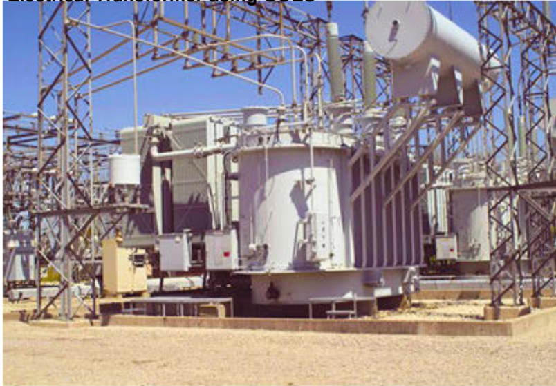
Figure I-4 Electrical Transformer using GOES
