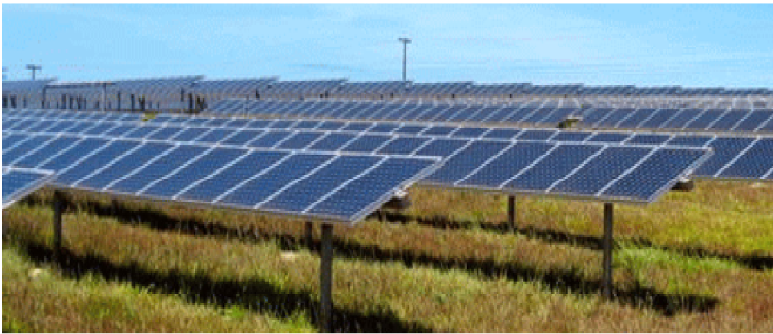
Figure I-13 La Ola PV plant, a utility CSPV system on Lanai, Hawaii
