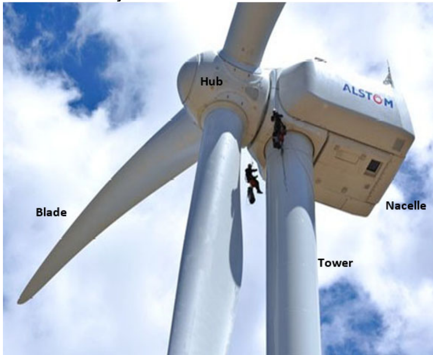
Figure I-1 Wind towers: Utility-scale wind turbine
