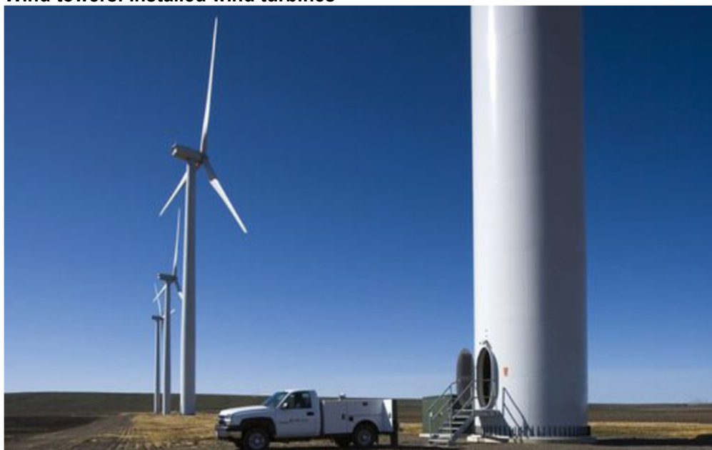
Figure I-3 Wind towers: Installed wind turbines
