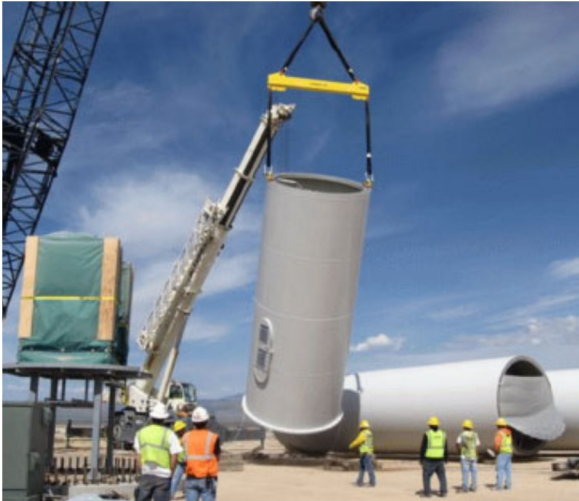
Raising the base section, with the foundation platform and power unit in the foreground.
