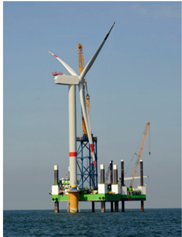
Installing the rotor assembly onto the nacelle.
