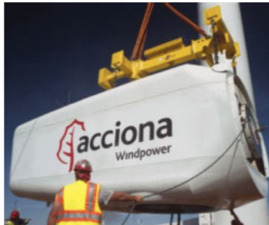
Raising the nacelle, containing the generator, for mounting onto the top-section flange.
