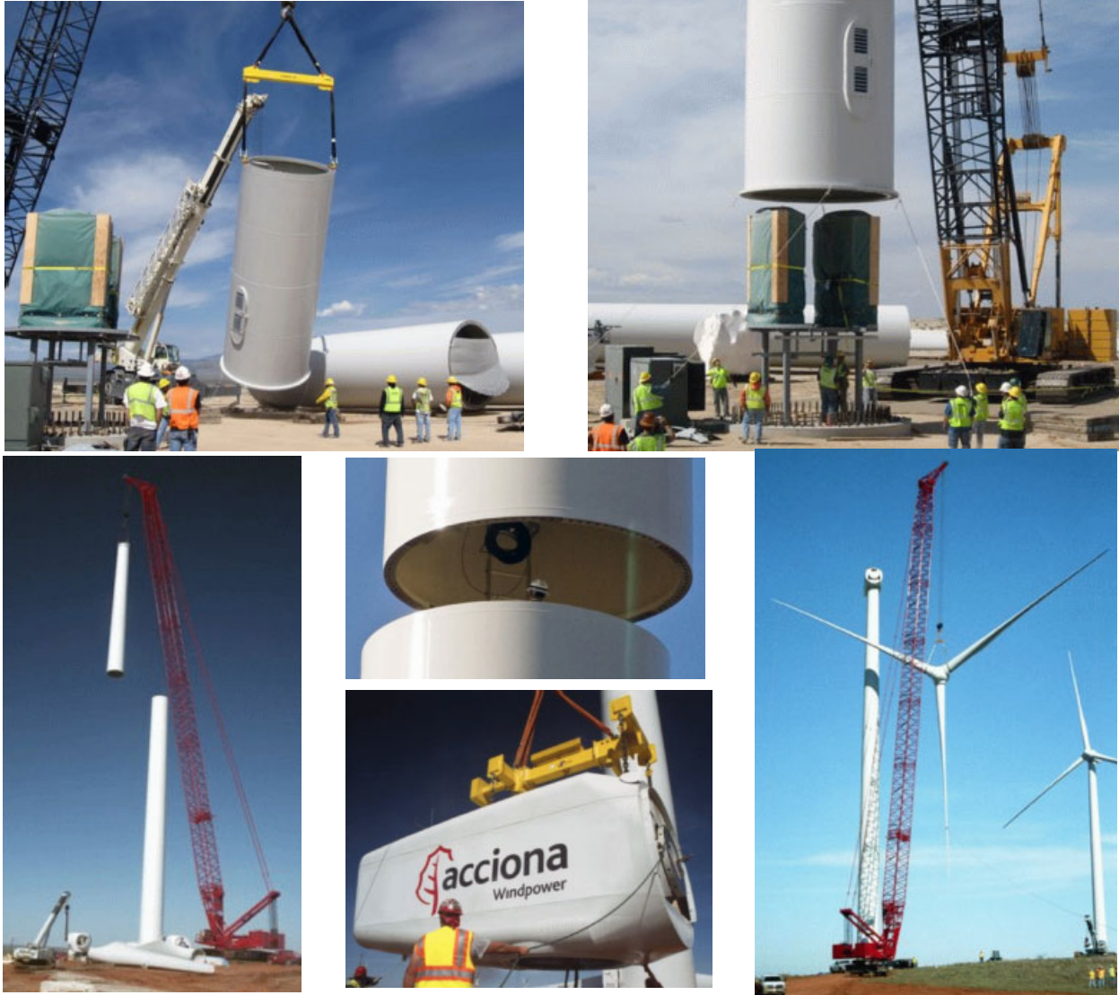
Figure I-7 Wind towers: Turbine installation
