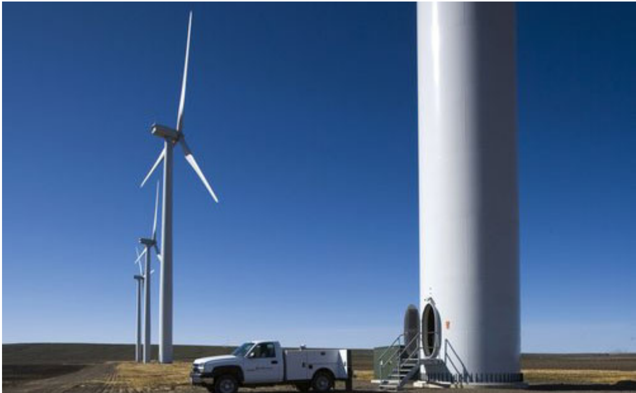
Figure I-3 Wind towers: Installed wind turbines
