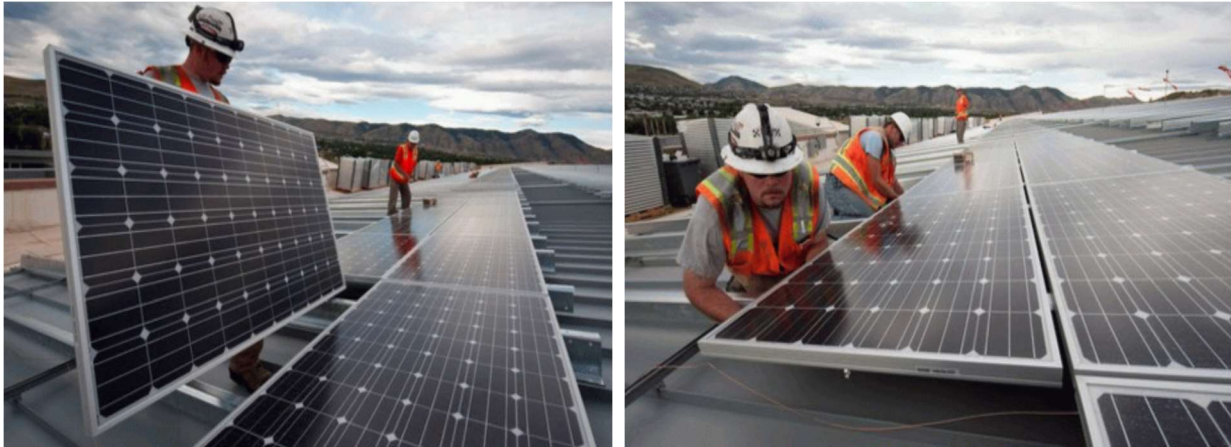
Figure I-11 Installation of a nonresidential CSPV system
