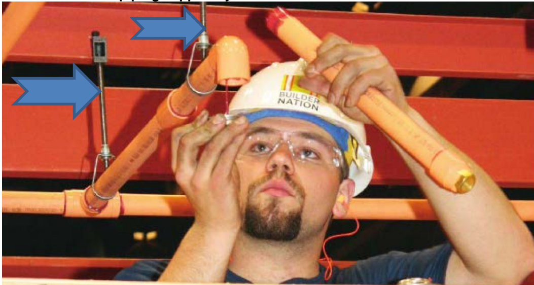
Figure I-2. Threaded rod in a piping support system
