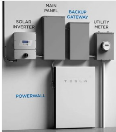
Figure 1 Example of an installed Tesla Powerwall and Backup Gateway
