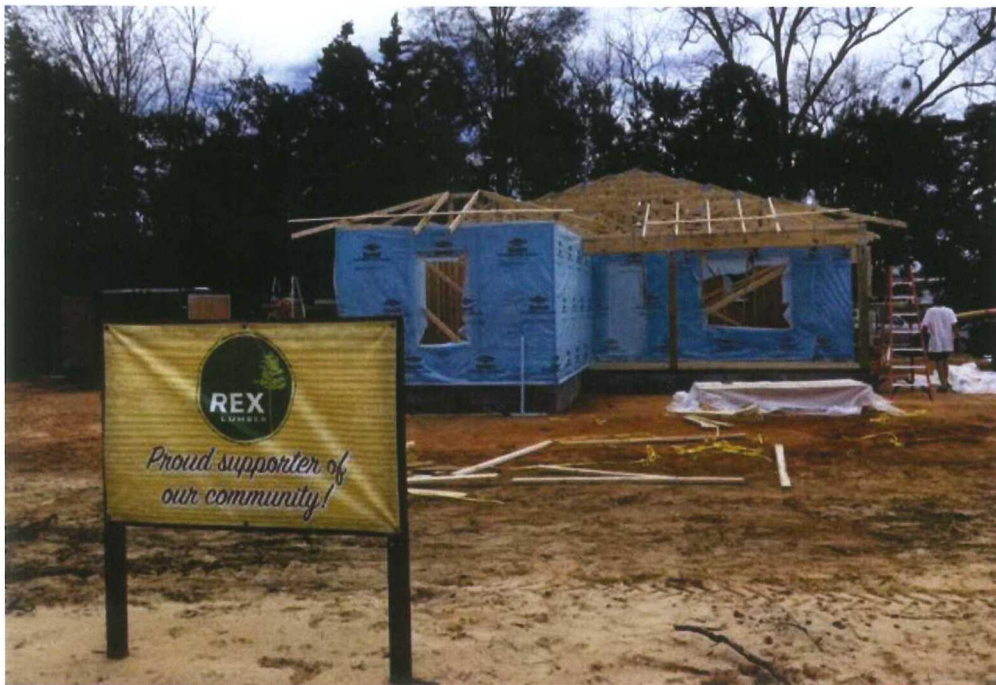
Graceville Home Under Construction
