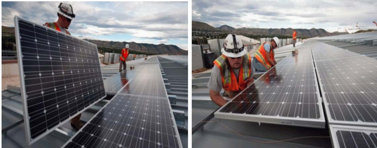
Figure I-14 Installation of a nonresidential CSPV system
