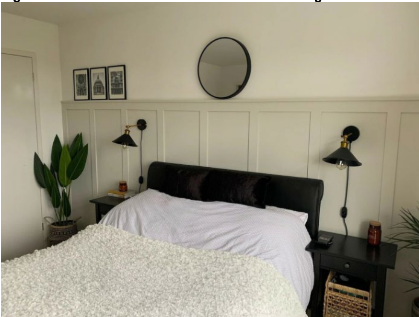
Figure 1.7 WMMP: Board-and-batten wall moulding
