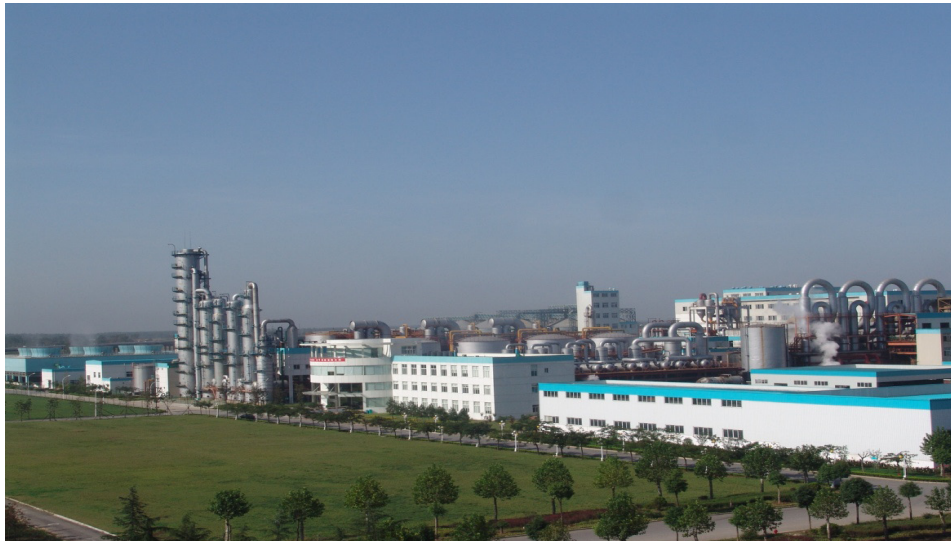
Figure 4. Henan Tianguan Enterprise Group Co., Ltd.'s commercial fuel ethanol biorefinery. The feedstocks are grain (corn and wheat), molasses, and cassava. Tianguan plans to upgrade this facility to produce bioethylene, biogas and biodegradable plastics. (Reprinted with permission from Tianguan.)
